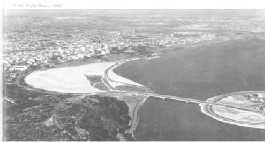
Figure 1: Filling in Mounts Bay for the Narrows Interchange, 1960s Note: the white patch in the image is the sand used for the project. (Source: http://www.cbcbg.org.au/projects/mounts_bay.htm )
